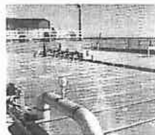
The Rolling Hills WRF Rated Capacity: 1.0 MGD Operating Mode: Batch SMU Type: Double Deck
